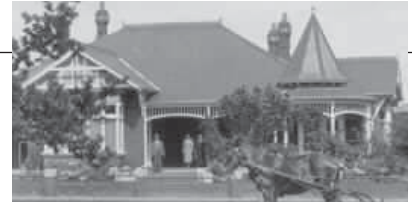
View towards Kingston Street, Malvern East (Reg No. 2499)
