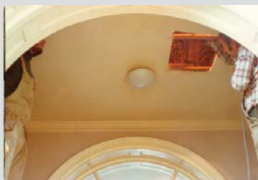
Detail of Northbrook ceiling c1980 Reg No17345
