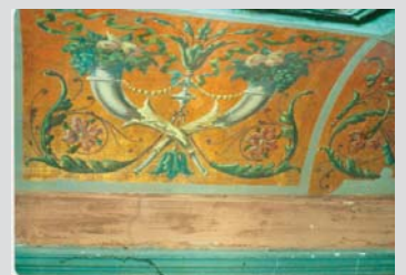
Removal of the Northbrook false ceiling c1980 Reg No17341
