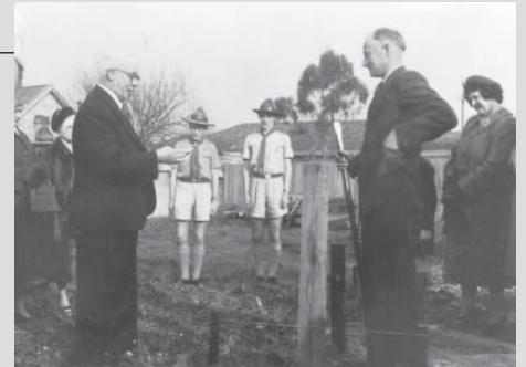
Bedding the first tree stump at 1st Malvern Scout Hall, 1953 Reg No 2159
