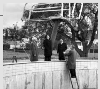
Construction of the diving tower 1969 Reg No 5357
