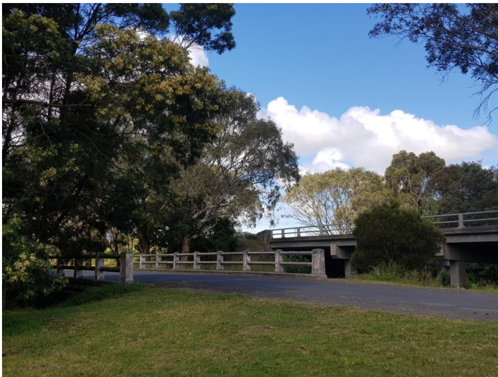
The 1939 bridge over the Tarra River with the Bicentennial Bridge in the background
