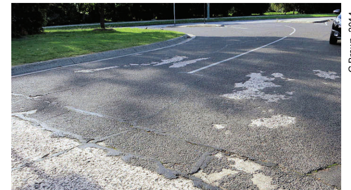
Worn bitumen reveals original concrete Pall Mall & Windsor Ave
