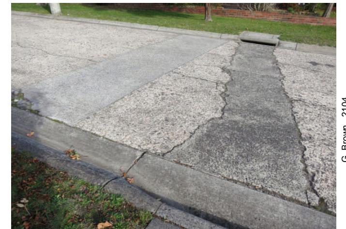
Different methods of road repair in Sherwood Rd
