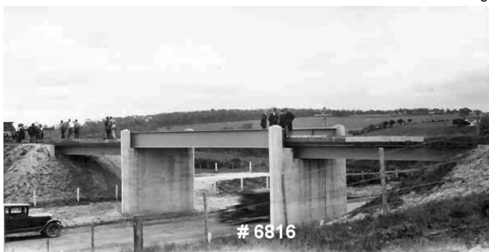
Inspection of the bridge across Warrigal Rd. Overhead power wires yet to be installed.
