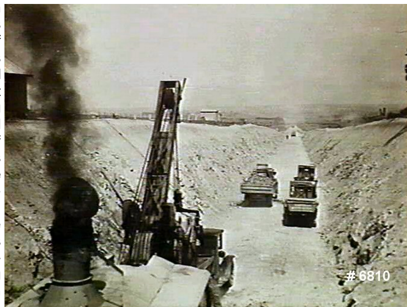
Excavation of the cutting with a steam shovel
