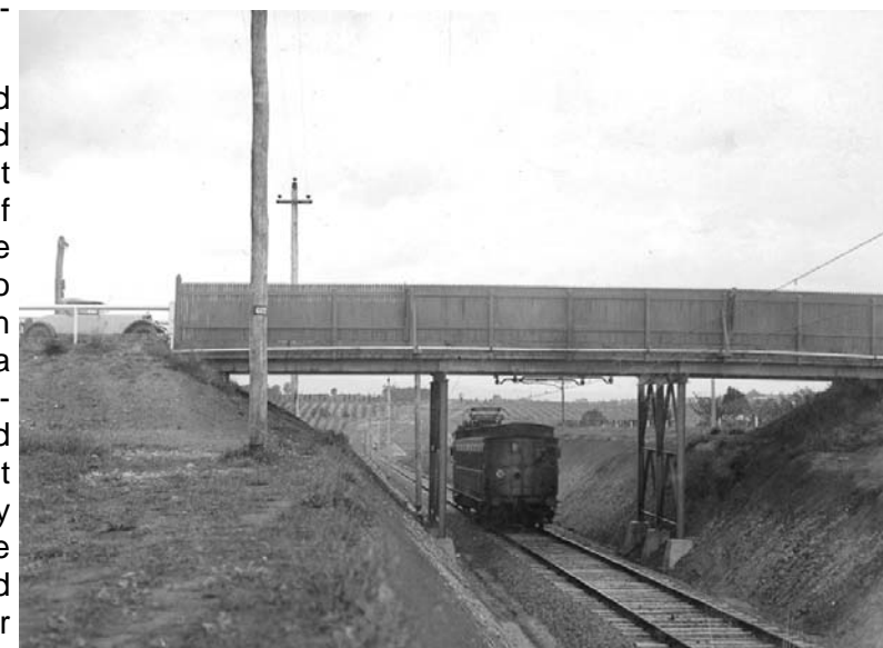
Lawrence Road Bridge, looking East
