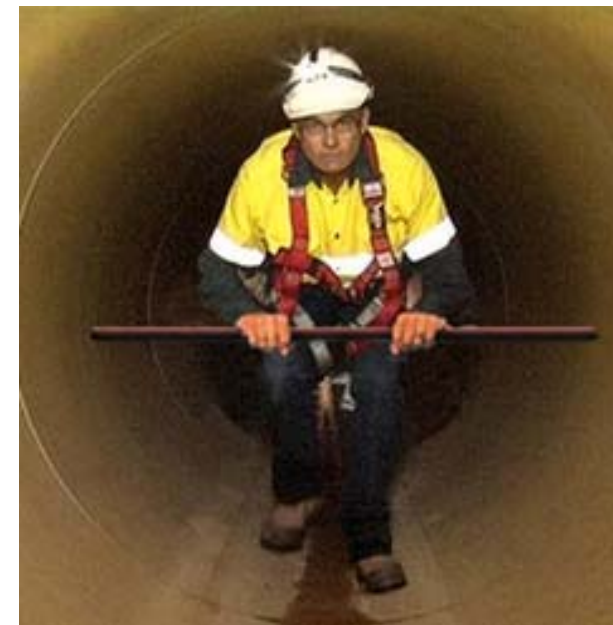
This picture, adapted from others, seeks to show how Laurie Ryan used a pole to help maintain his balance while searching a large sewer for flood damage after heavy rain. Nowadays a robot camera is used to inspect sewers for damage.
