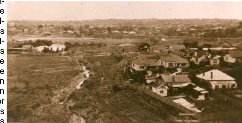
A view from the recently installed power pylon looking over Kooyong Koot on Gardiners Creek towards Saxby Road, Glen Iris C.1925.
