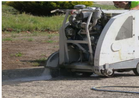
Using a circular saw to cut the roadway from the kerb
