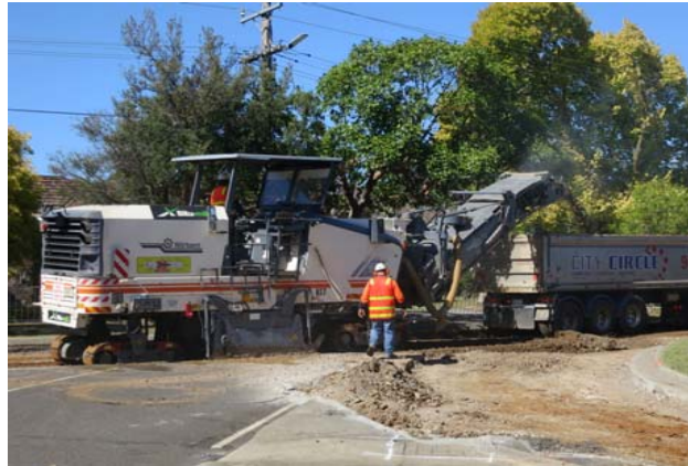
Excavation and removal of the old roadway
