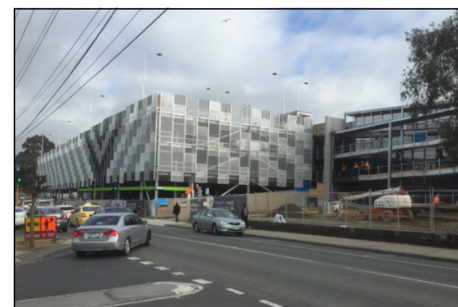
The carpark looking NW. Coloured open mesh cladding installed
