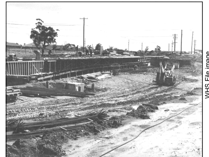
Looking NNE at what is to be the crossing over the Monash Freeway/Arterial road. Reinforcing and concrete formwork being erected. A shopping centre and Golden Fleece service station are in the right background.
