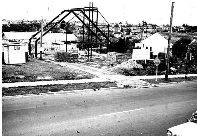
Syndal Baptist Church Sanctuary during construction at 588 High Street Rd (1968) with Church Hall at the rear.
