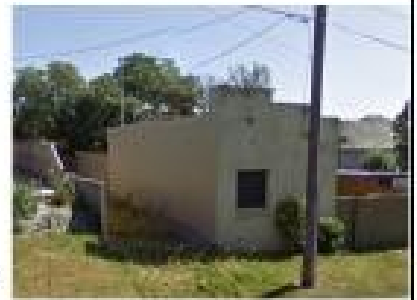
The solid brick Gallus dairy shop
