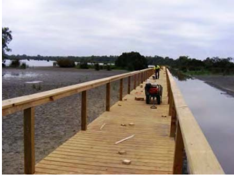
Board walk progressing well
