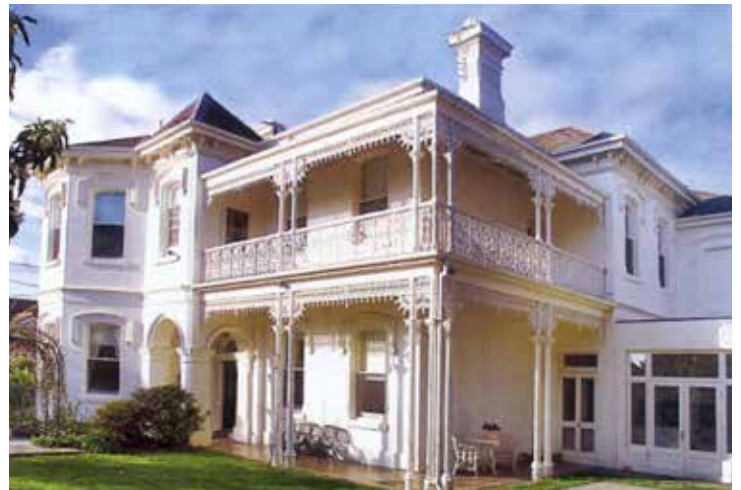
'Carrington' 58 Kooyong Road Armadale (undated) Stonnington History Centre MP14987
