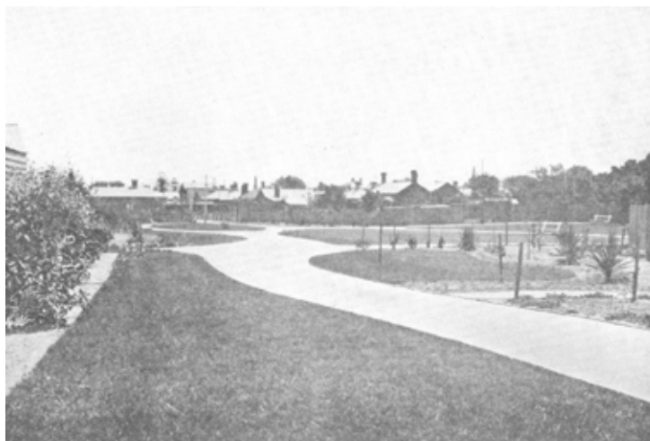
Gladstone Park in Windsor c1913, created from the former easement for the old St Kilda-Windsor railway loop line (1859-62) Published in Prahran City Council annual report, 1912/13 Stonnington History Centre PH9171
