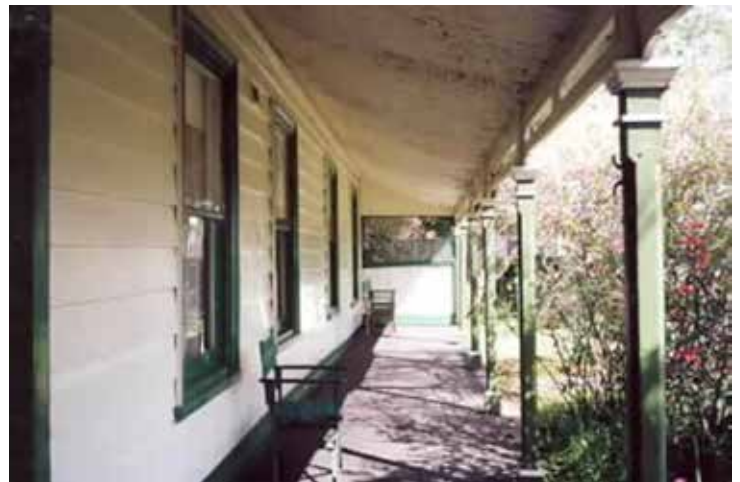
Glendearg, former Wattle Tree Hotel, 196 Wattle Tree Road Malvern 1990. Image: Di Foster Stonnington History Centre MP8274
