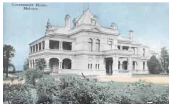
Stonnington, Government House Malvern c1910 Stonnington History Collection MP1115
