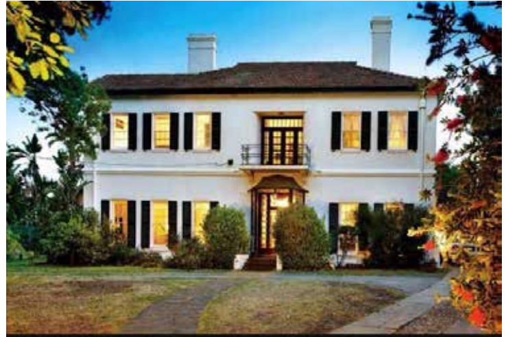
6 Haverbrack Avenue Malvern 2008
