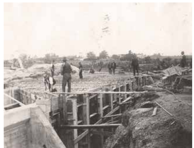
Placing deck reinforcement Scotchman’s Creek 1924 (Irwin Collection)
