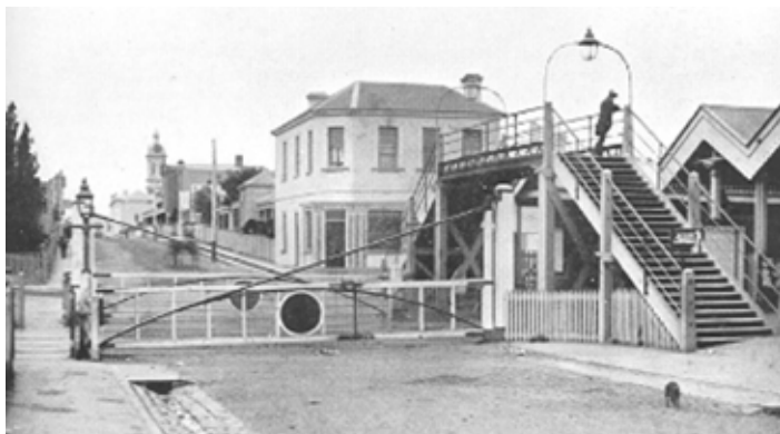
Greville Street Prahran 1867. The photo was taken looking east and shows the railway station and the Railway Tavern. Stonnington History Collection PH13125
