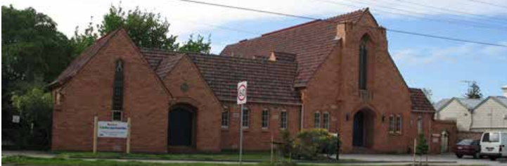
Ewing Memorial Church hall and kindergarten (M.Chestney 2006) Stonnington History Collection SHC60435
