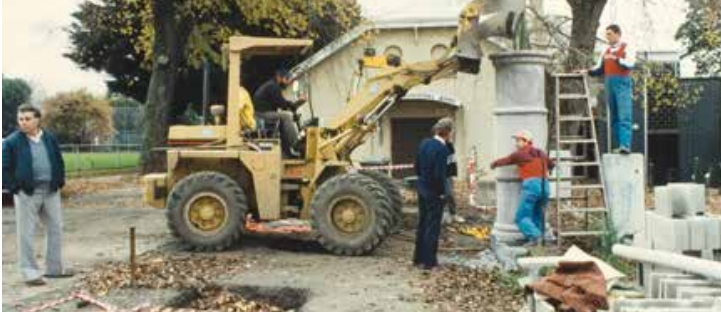
Construction of the Northbrook Art Garden 1989 Stonnington History Collection MP 9326
