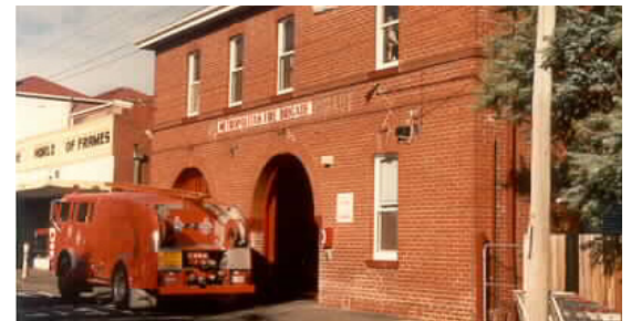
Fire Station, Willis Street Malvern 1988 Reg no 7307
