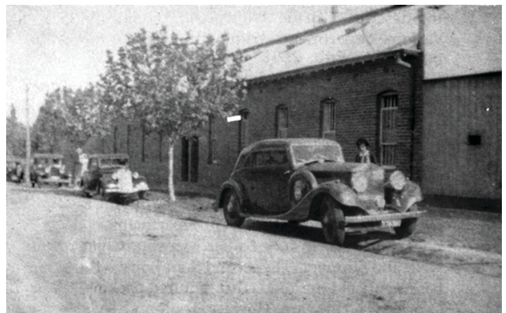
Gilpin's warehouse Belson Street East Malvern c1934 Reg no 62048
