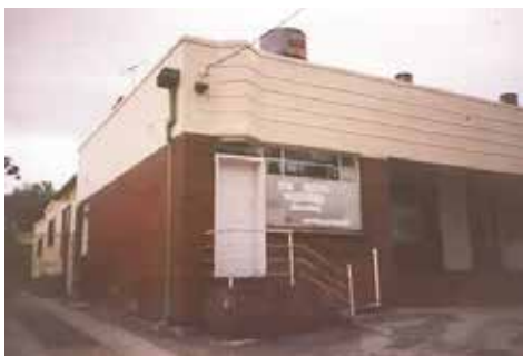
The Old Dairy, Tooronga Road, Malvern East 1994 prior to its demolition. Reg No 8057
