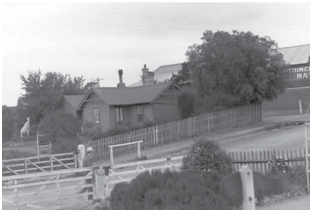
Gatehouse close to Gardiner Station, Burke Road, Gardiner 1917 Reg No 2686
