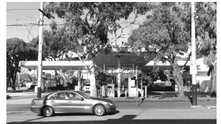
South west corner of Malvern and Glenferrie Roads, Malvern 2015
