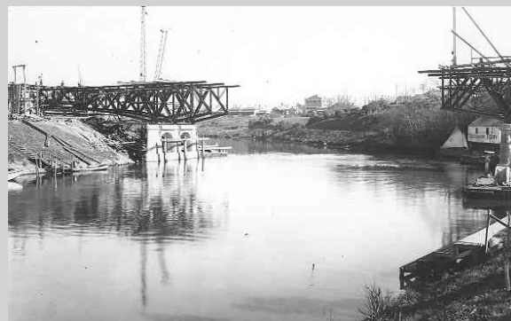
Construction of MacRobertson Bridge c1934 - Reg No 10061
