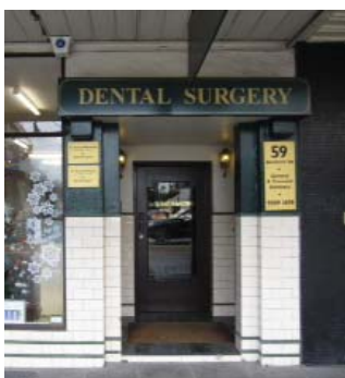
Entrance to 59 Glenferrie Road Malvern 2013
