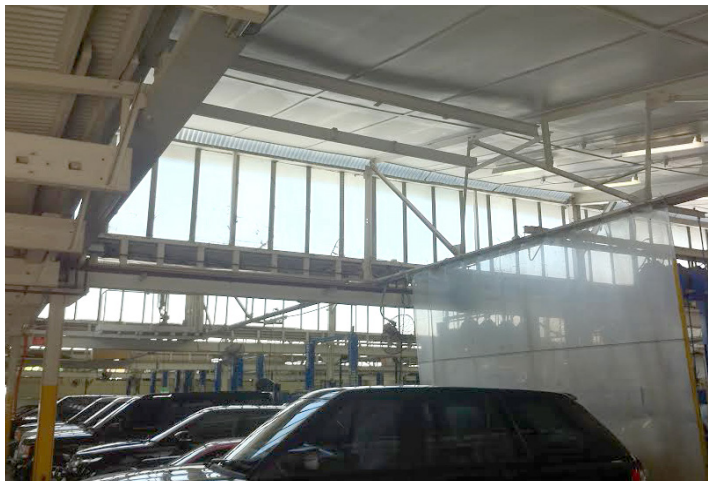
Interior 1305-1315 Malvern Road Malvern, 2013
