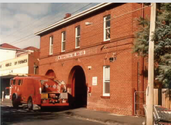
Malvern Fire Station Willis Street Reg No 7307
