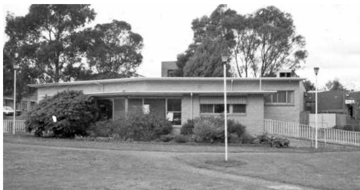
R. G. Moss, Library, Bowen Street Chadstone (Malvern East) 1985 Reg No 12136
