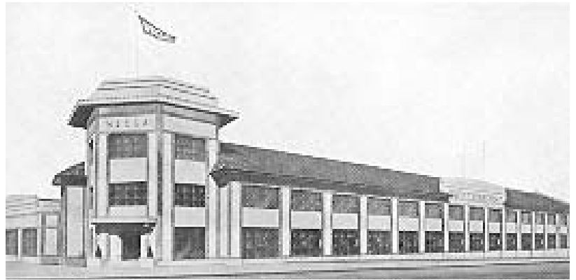
Hecla Works Chapel Street North, on the east side of Chapel Street, north of Toorak Road 1927 Reg No 12707
