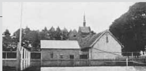
The original 1858 school, close to St George's Malvern Pre 1925
