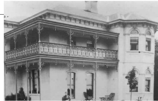
Kelmescott, Huntingtower Road, Armadale 1900 Reg No 5208
