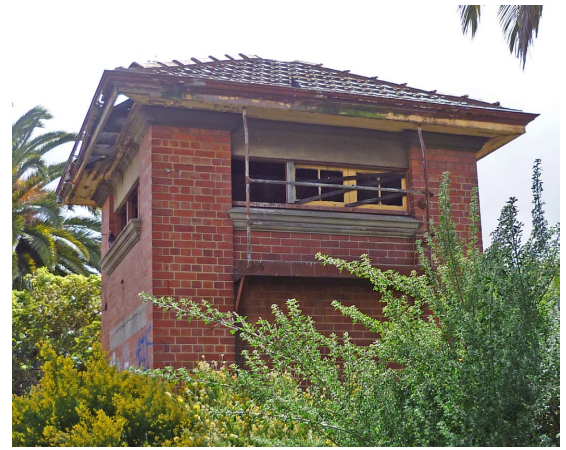
Brick Tower Toorak Station 2011
