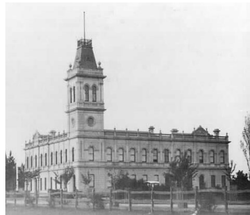
Exterior view of the Malvern Shire Hall 1886 Reg No. 677
