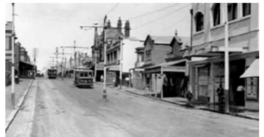
High Street, east of the railway overpass 1915 Reg No 8772
