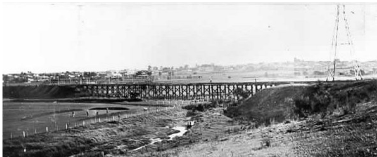
Black Bridge over Gardiners Creek looking west from Ashburton to East Malvern c 1930. The Black Bridge -a single line timber trestle bridge spanning Gardiners Creek, and later the Glen Waverley Railway, was constructed in 1889 for the Outer Circle Railway. It was removed around 1938 Reg no 5092
