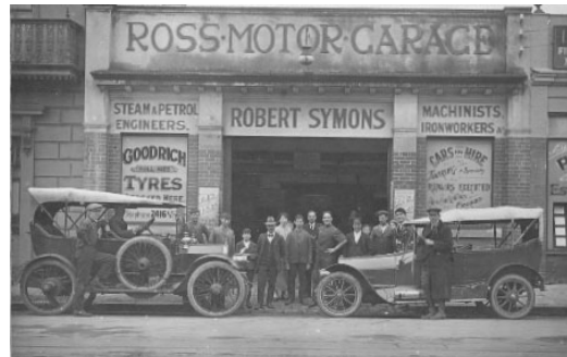
Garage, 449-453 Toorak Road, Toorak (east of Wallace Avenue) c.1920 Reg No 23425
