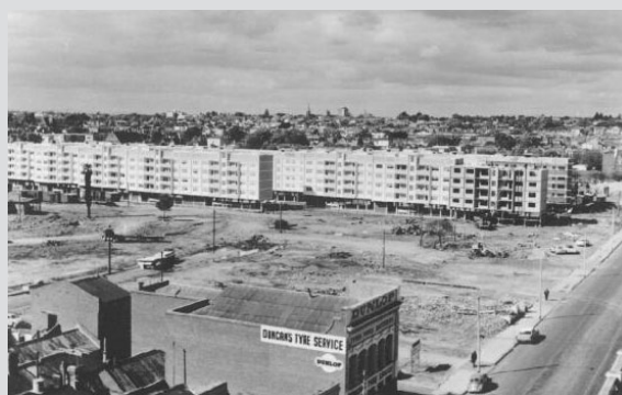
Construction of 'walk-up' flats on the Horace Petty Estate, April 1965, looking east along Malvern Road. 1965 Reg No 6067
