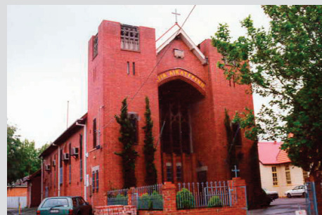
St Catherine's Greek Orthodox Church (Former Peace Memorial Methodist Church), Epping Street East Malvern 1994
