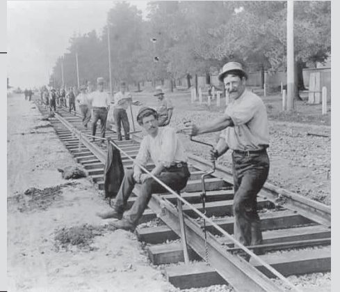
Laying tram tracks in Dandenong Road Armadale Reg No 1911
