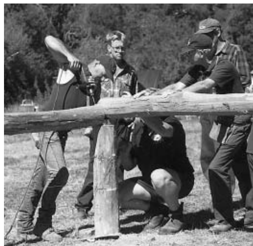
The Friends of Wonnangatta Valley working on a replica of the original post and rail fence around the old stockyard at the Homestead site. The materials were brought in by the Friends.
