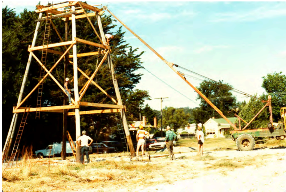
Erecting the Poppet Head on a warm Summer day in 1982. Ron Nicholls's heavy truck was very important. All done without the need to apply for a planning permit!
