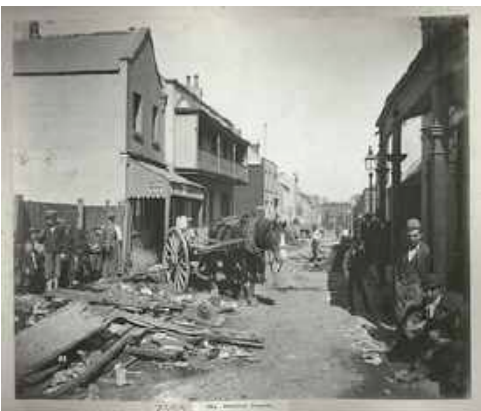
Hunt Street, Sydney. Cleansing of homes and destruction of waste near Haymarket demolished
