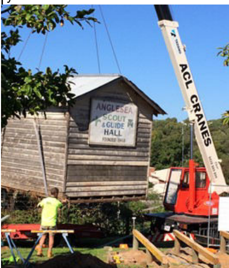
Bathing Box being craned into position at History House
