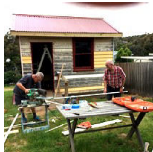
Keith Hornibrook and Kevin Pollard work on the Bathing Box
