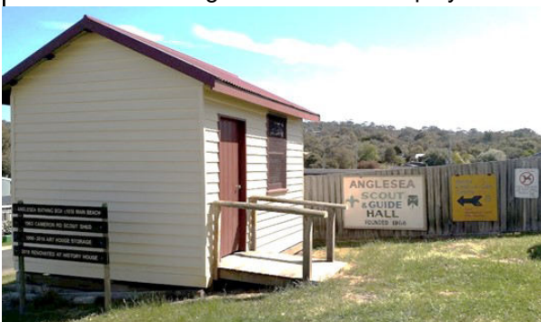
The fully restored Anglesea Bathing Box
