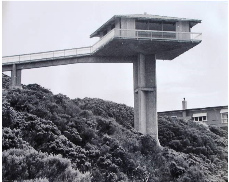
A 1978 photo by the Herald Newspaper, of the Pole House
