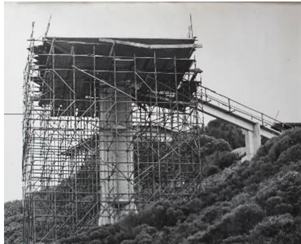
The final concrete pour, showing the extensive scaffolding
