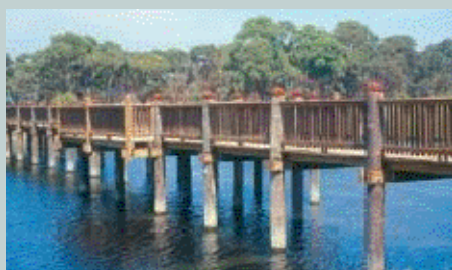
Laverton Creek Bridge
