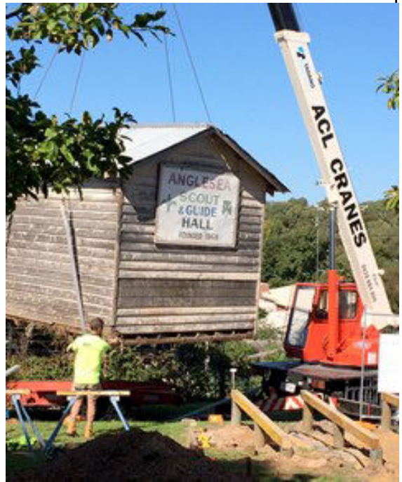
The Bathing Box is craned into place.
