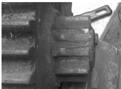
Damaged Cast Iron Gear Teeth
