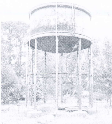
The 20,000 gallon water tank beside the Birregurra Station, provided water for the steam
