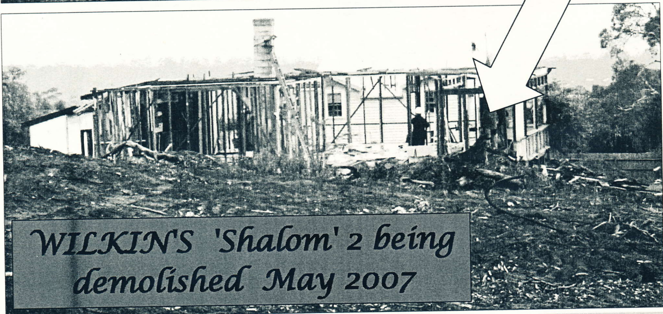
Shalom No2. was demolished during May 2007. Land re-subdivided
