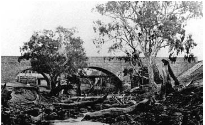
Bluestone Bridge open 1867 by Duke of Edinburgh
